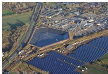
Construction of the large thermal storage during 2014
