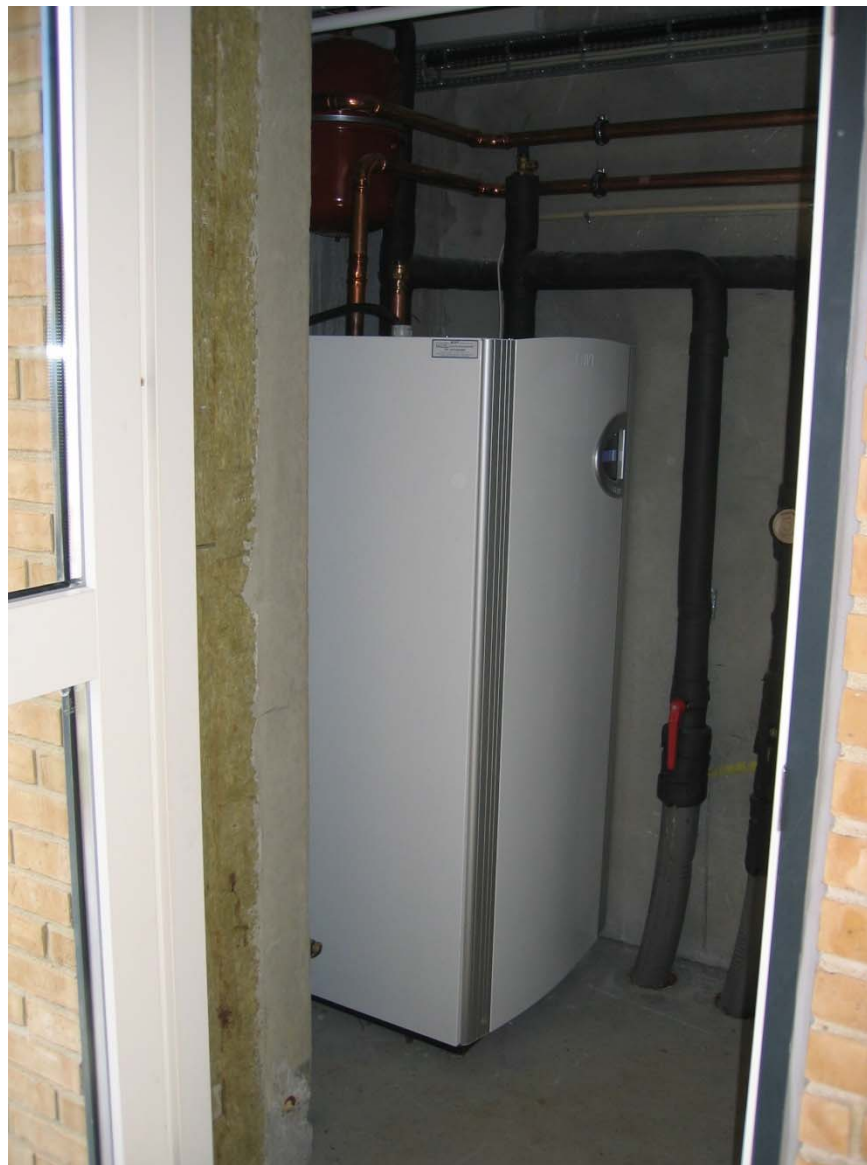
Buffer tank for shared heat pump
